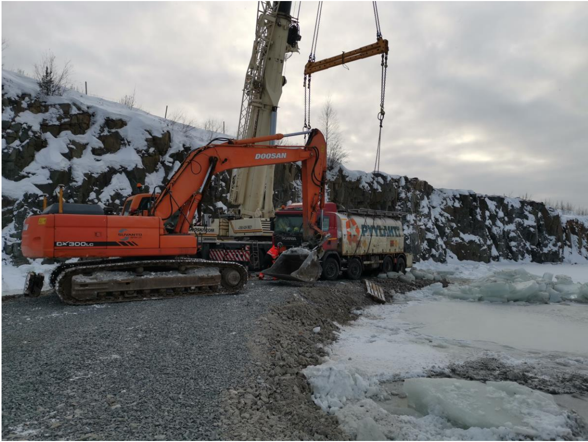
Lifting operation done
