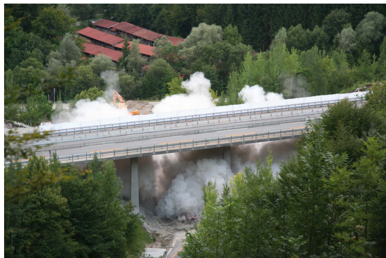
Fig. 8a - 8c. Blasting the southern bridge
