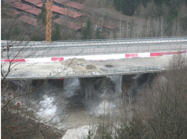
Fig. 10b - 10c. Blasting the northern bridge
