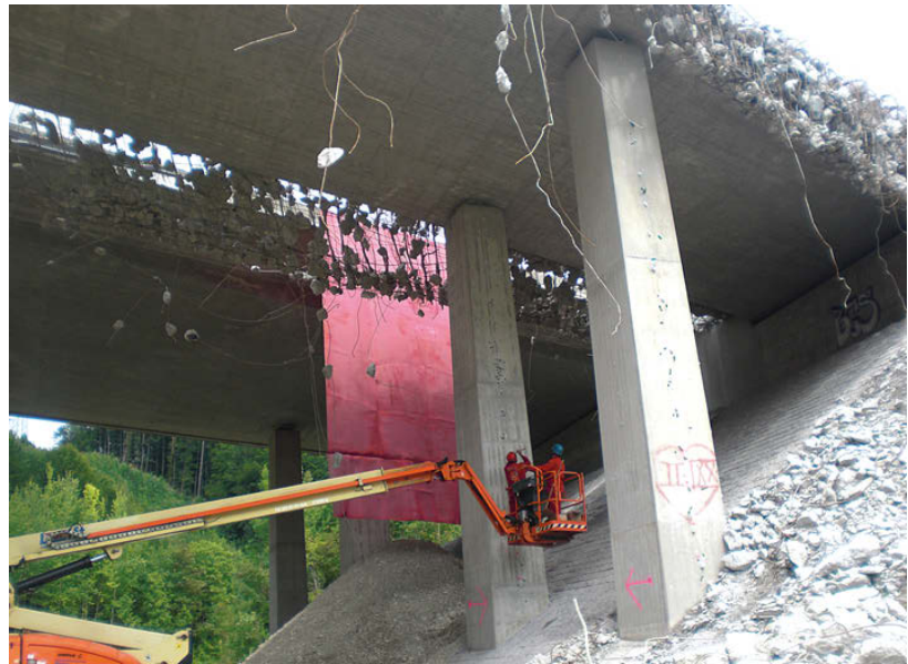
Fig. 6. Charging pylon 1
