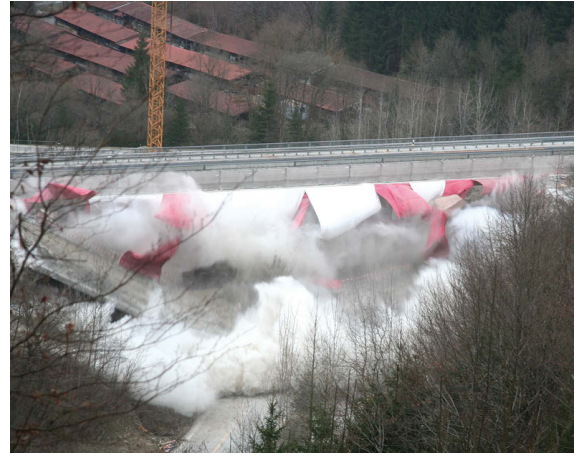
Fig. 10b - 10c. Blasting the northern bridge
