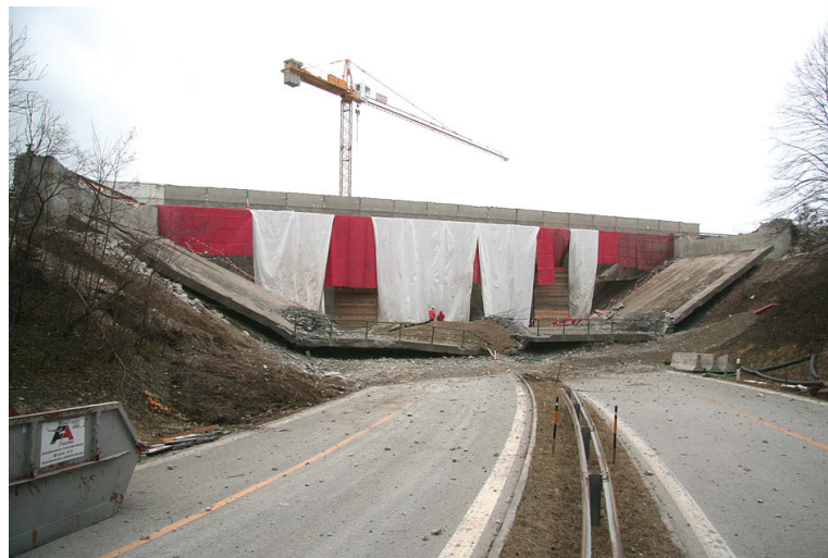
Fig. 11. Northern bridge, blast results
