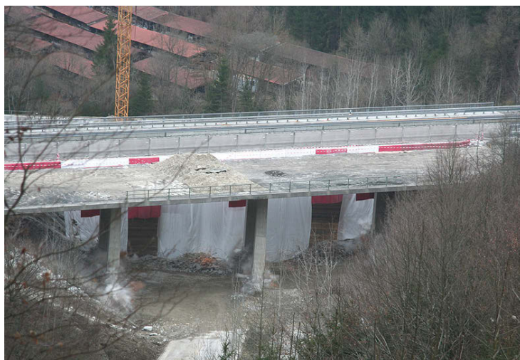
Fig. 10a. Blasting the northern bridge
