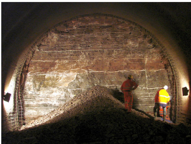
Fig. 26: Position of the muck pile after blasting on 23 March 2016 at about 11.15am
