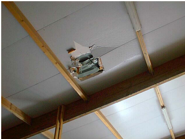
Example 2: Damage to a factory roof and blocks landing approximately 200 m in front of the blast
