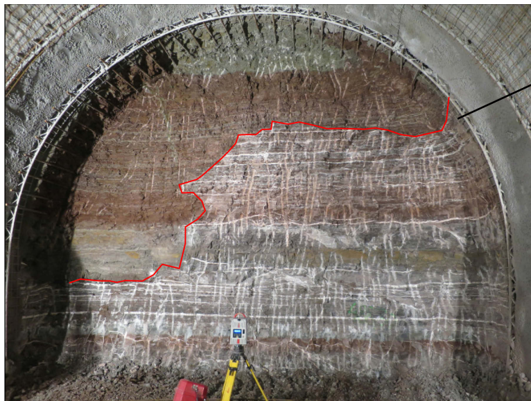
Fig. 8: Example of a tunnel face in the roof section with irregular leaching of the gypsum in the interbedded strata of calcareous clay-siltstones
