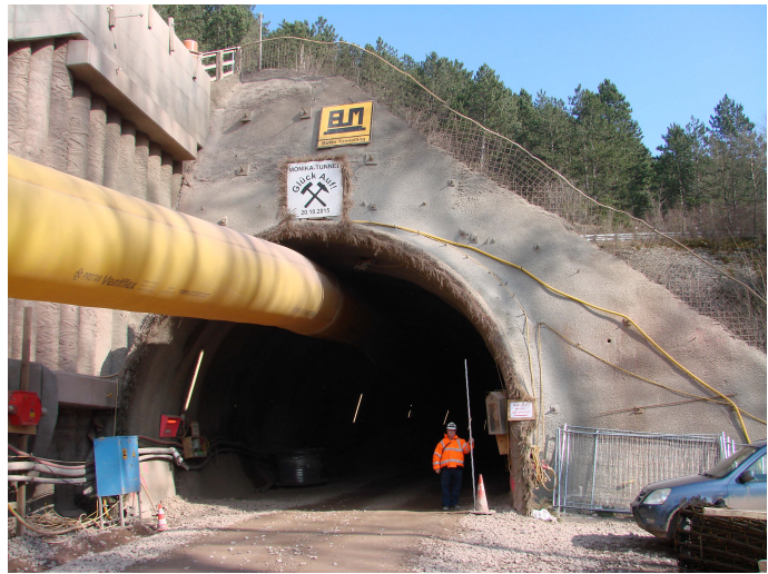
Fig. 2: West portal of the new Zierenberg Tunnel ('Monika Tunnel') alongside an embankment reinforced with bored piles
