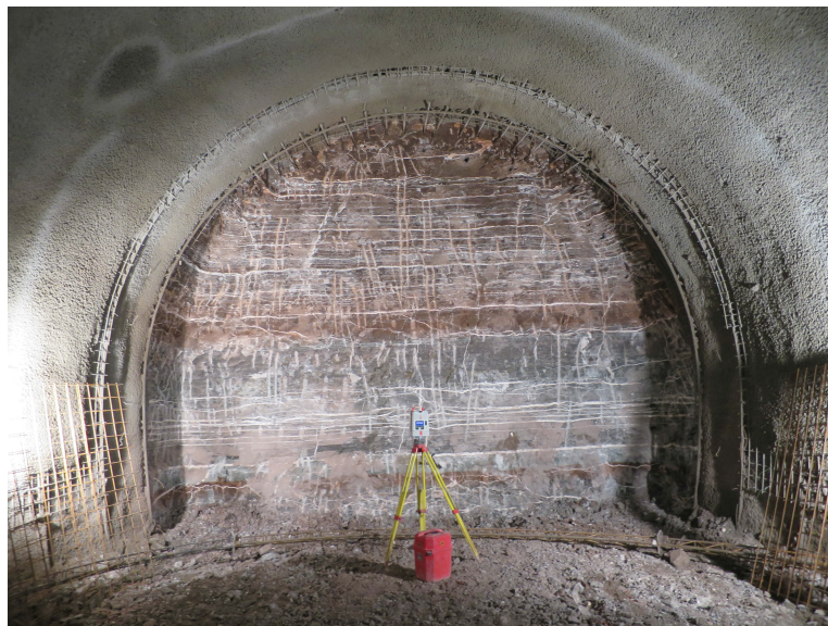
Fig. 9: Example of a tunnel face in the roof section with unweathered, calcareous, highly gypsified interbedded clay-siltstones with layers of fibrous gypsum
