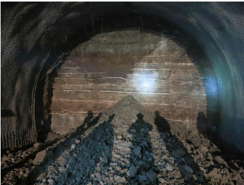
Fig. 25: Position of the muck pile containing small rubble after the first blasting on 8 January 2016
