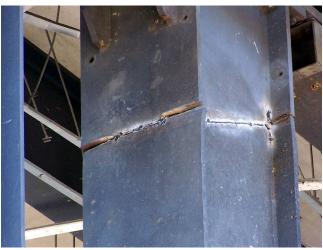
the application of 292 shock-tube detonators is not appropriate for such an operation. The tolerances of the delays may have led to the cut-offs.
