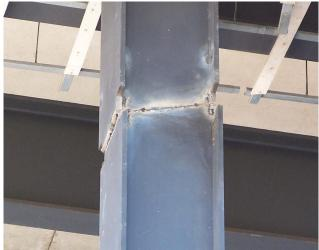
Fig. 6: improper cut
